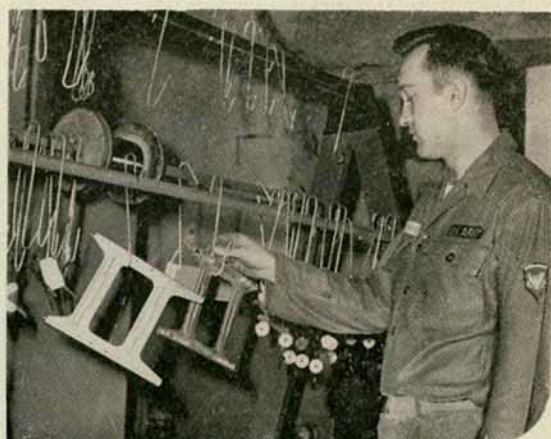
Metal plating for activities throughout USAREUR is carried on at three TASCOM installations—Saumur General Depot, Verdun General Depot, and Pirmasens General Depot. Most of the plating is done on parts to be used in military radios, microwave sets, and teletype machines. Here a metal plating specialist puts pieces on the finishing rack.
